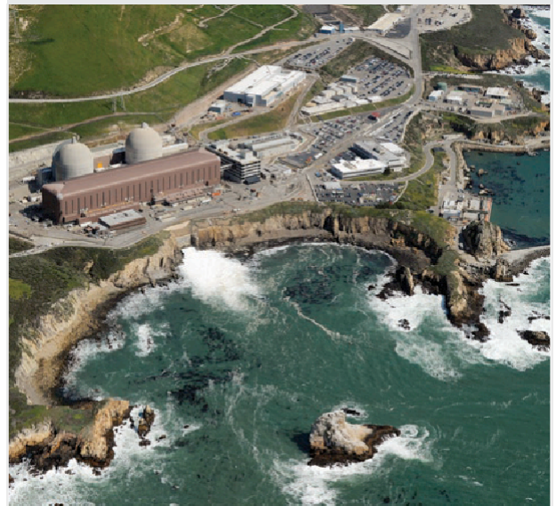
FIGURE 12: The Diablo Canyon nuclear power plant in San Luis Obispo County
