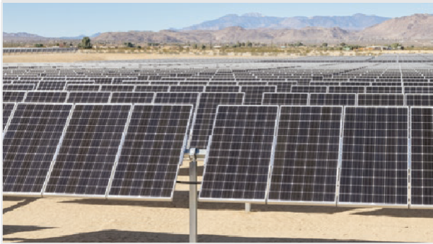
FIGURE 13: The Topaz Solar Farm in San Luis Obispo County is a 550-megawatt photovoltaic power station, one of the world's largest solar farms.
