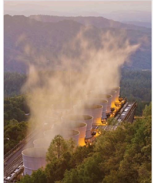
FIGURE 15: The Geysers geothermal power plant is the largest producer of geothermal electricity in the world
